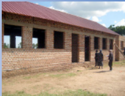
Bufasi Primary School under construction CFTC UCOBAC CDP 2013
